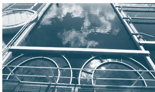
Installation with two Z4000 FlocBees operating in parallel, a good solution in wide tanks.
