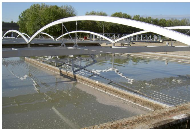
The scraper blade is fixed to a sledge which is propelled step-by-step by the drive bar. The sledge changes its direction of motion at each end of its travel. This allows several interacting sledges with scraper blades to be used in the same tank. For the return movement, the scraper blade swings up to avoid the sludge.
