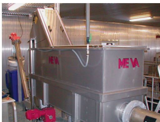
Meva Monoscreen in combination with a Screw Wash Press
