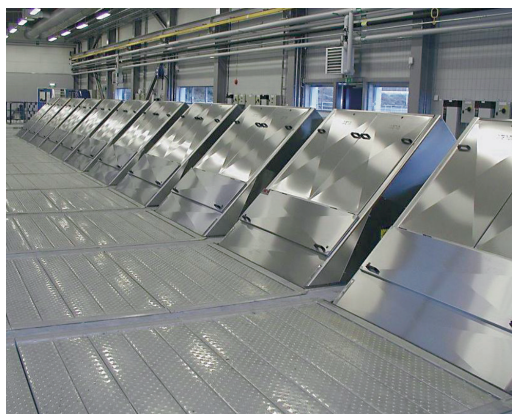
Meva Monoscreen in a WWTP
