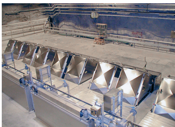
Meva Rotoscreen in a WWTP
