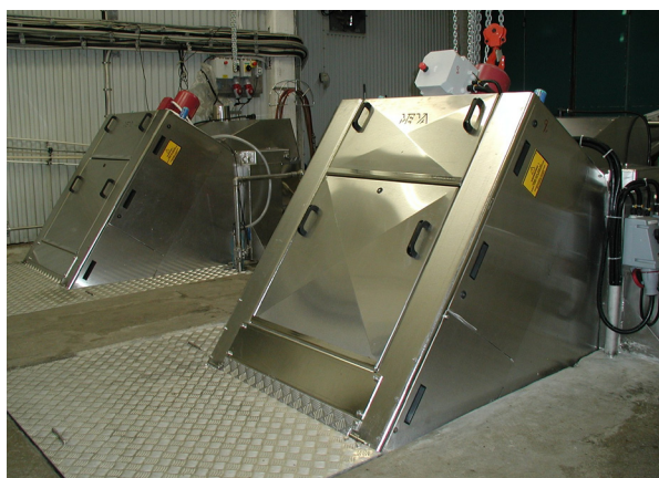
Meva Rotoscreen fully enclosed
