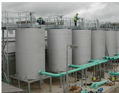
Installation of Lamella Settlers and six 19m³ flocculation tanks in the UK
