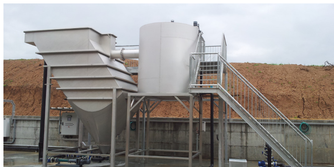
Lamella LS is a Lamella Settler with sludge thickening bottom hopper
