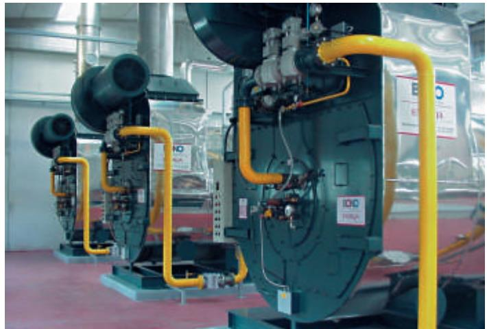
**STEAM-MATIC SG boilers offer superior performance:** the innovative design of the pressure vessel ensures excellent heat transfer in two passes and provide full accessibility to the boiler and the flue gas reversing chamber. The large volume of water and a wide steam chamber provide high working flexibility and a considerable steam reserve.
